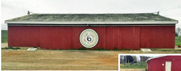
Footers are in place
