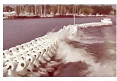
violently rock harbored crafts. The recommended wave attenuator, WhisprWave® is designed to extract the energy from incoming waves. Anchored to the river bottom they would be used 9 months and removed and stored during the winter.
